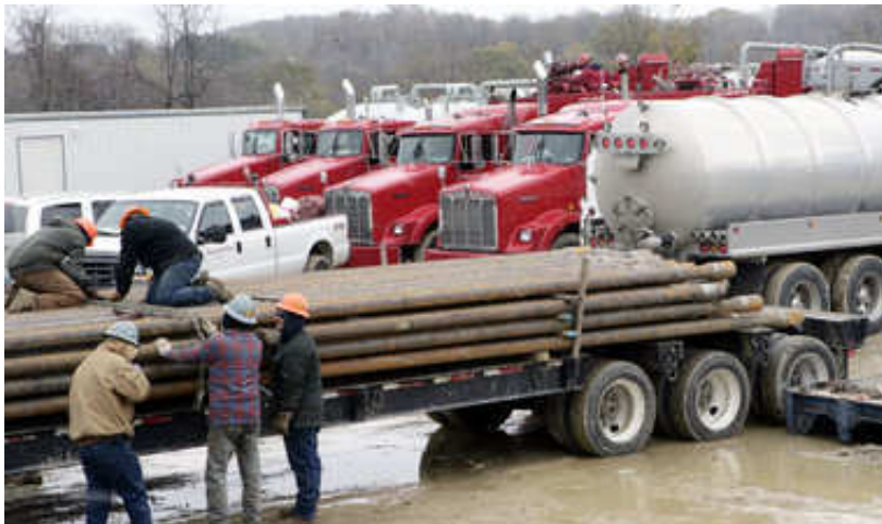
Workers stack the steel shafts, used in drilling wells thousands of feet into the earth to get to the Marcellus shale, on a farm in Houston, Pa. (AP Image)
