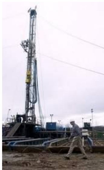
Gas drilling by Cabot Oil & Gas in Dimock, Pa., Thursday, November 5, 2008. Kenneth Komoroski walks by a drilling rig. (File photo)
